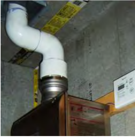
Figure 31. PVC venting on condensing tankless. Photo Credit: Noritz
